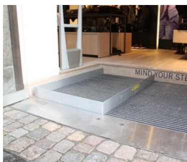
Safety plates in up position
